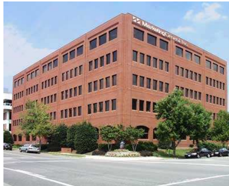
NRI BHPMS Office Building
